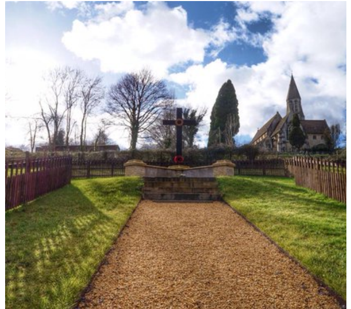
The cross after restoration 2014. The figure of Christ has long since disappeared and has been replaced by a ceramic wreath.
