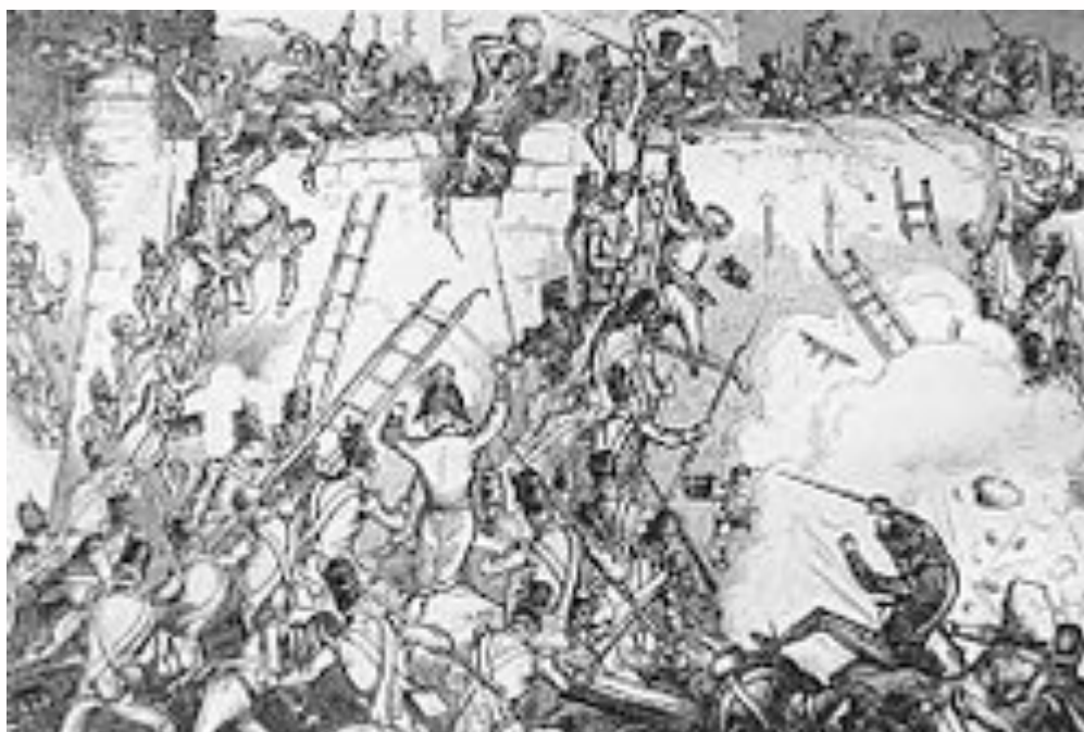
Picton's 3 rd Division manage to reach the top of the walls of Badajoz
